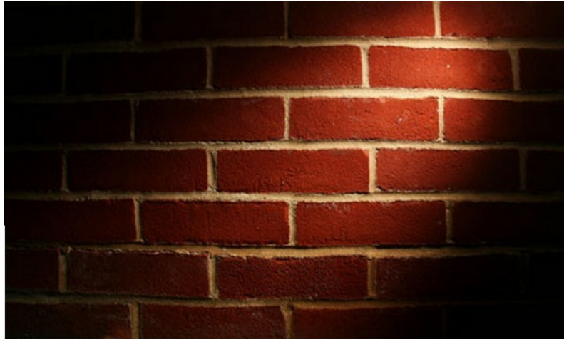
Beyond bricks: one compelling defence of buildings is the basic human urge to congregate. Photograph: Graham Turner for the Guardian
